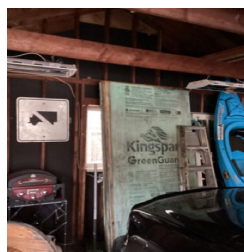
There was limited access to windows in the Detached Garage.
