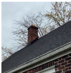
Roof of the Home
