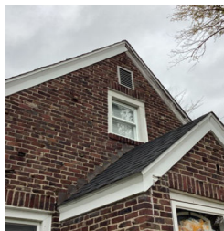
Roof of the Home
