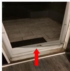
Front door screen door has a screen at the bottom is come detached.
