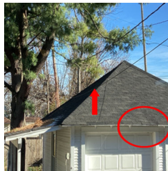
The garage has a sag on the front side, and a low hanging wire.
