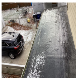
A railing is missing on the Balcony.
