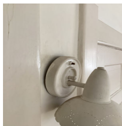
Light fixtures are detaching in the Upstairs Bedroom left of the master bedroom .
