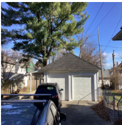
The Garage is shared with the neighbor.
